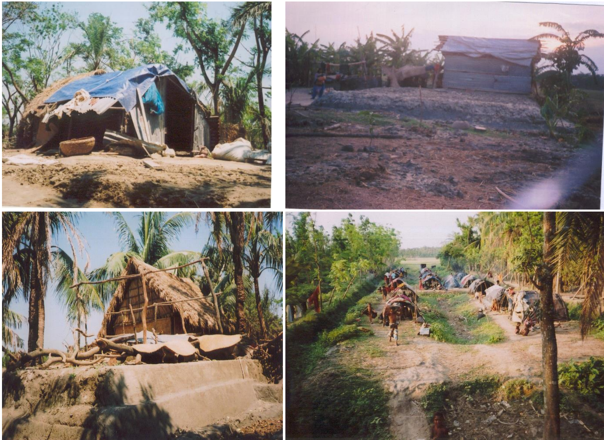
Figure 2 Devastation to houses and the type of temporary houses after Cyclone Sidr in 2007 (Source: the author).
