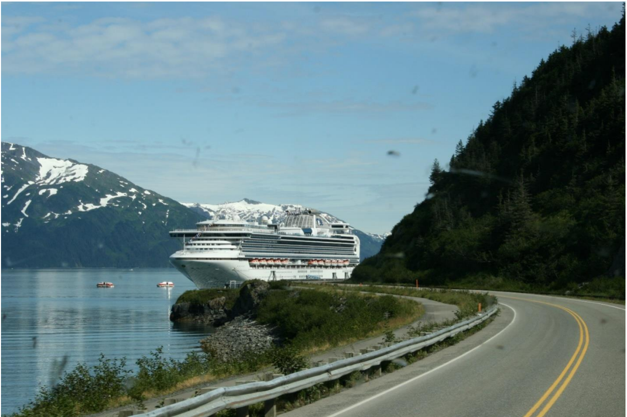
Figure 6 Sea Level rise imperils roadways
