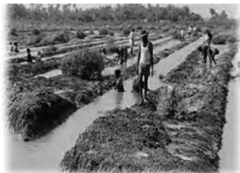
Before restoration of Mangroves - 1998
